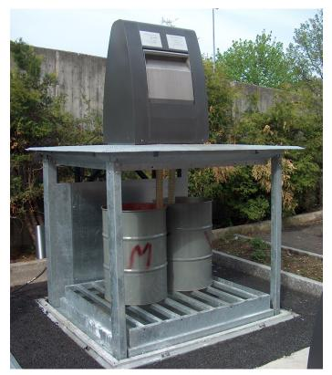
Collection Point for used oil with two barrels à 159 l
